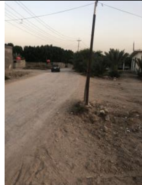
Current Situation at Al Thawiher Village
