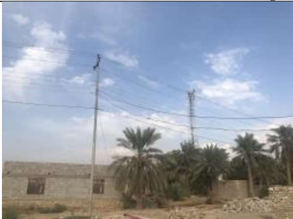
Current Situation at Al Tawawreh Village
