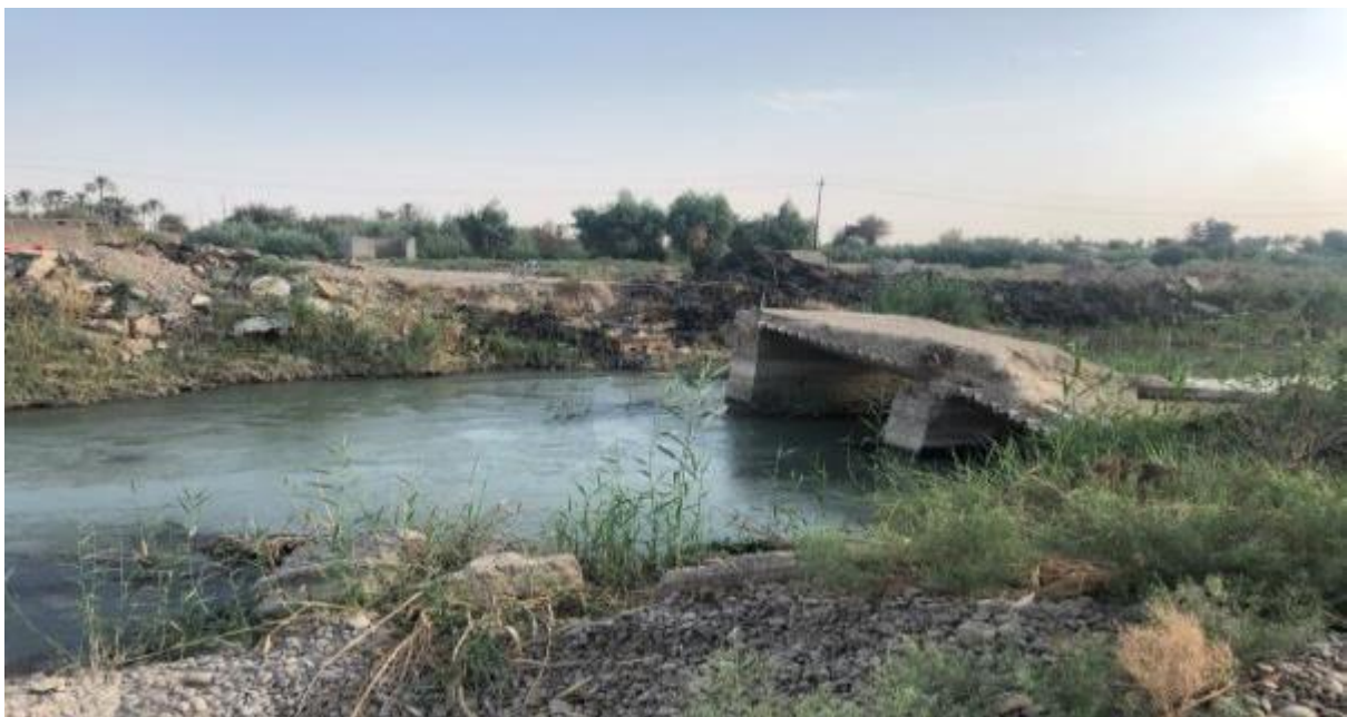
Figure 4: Photo of the current Culvert in Gewizrat village
