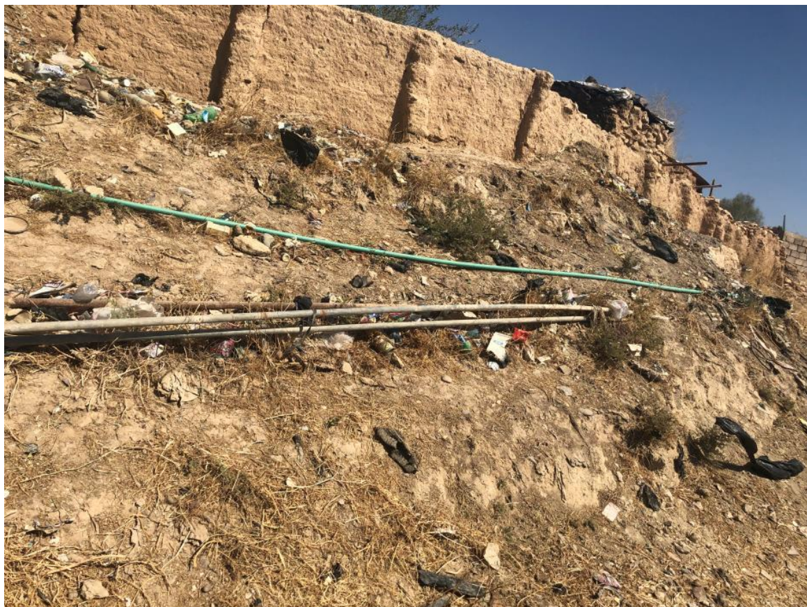
Current Situation of the water distribution network at Al Khanokah Village
