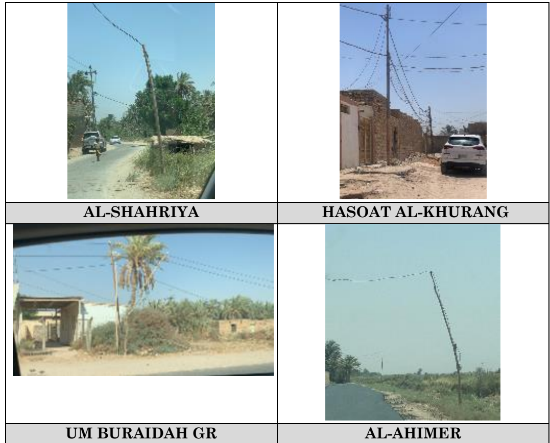
Figure 2: Current Situation at these Villages
