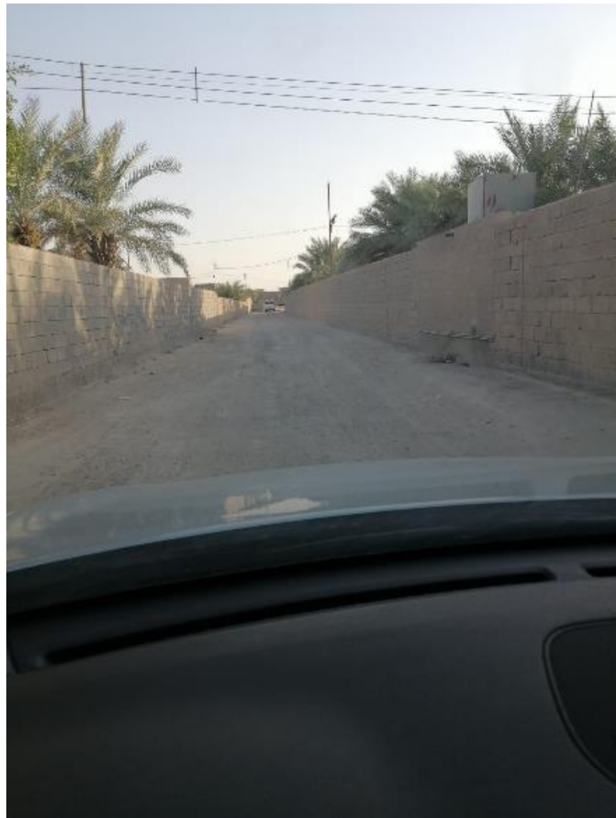
Figure 2: Road in AL-ASRIA Village
